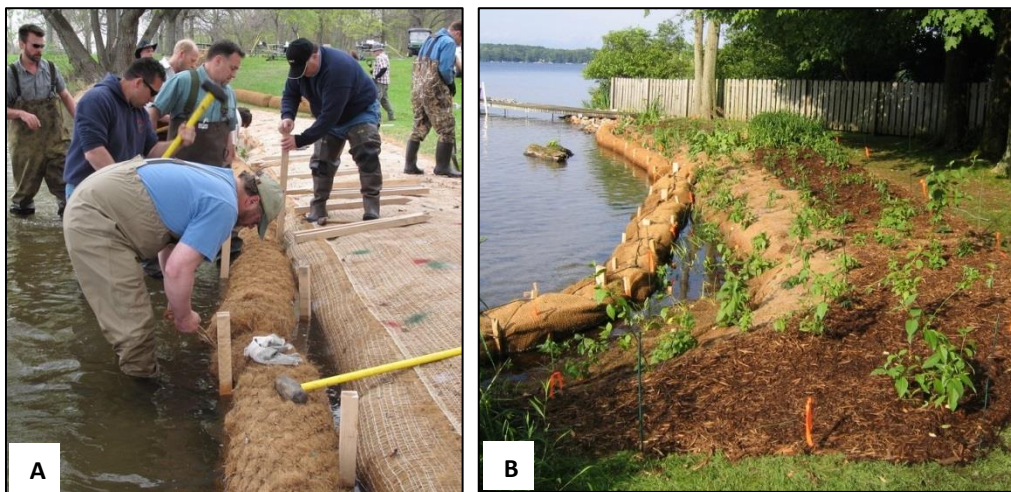
Figure 5.4: Installation of coir logs on Kent Lake, Oakland Co. (A), and a few weeks after installation of erosion blanket and brush bundle (B) on Gull Lake, Kalamazoo Co.
